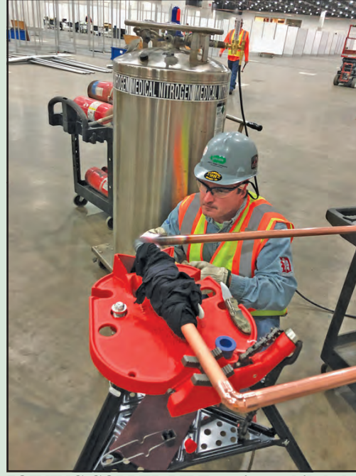
JOINING COPPER PIPE sections while helping put together the field hospital at the TCF Center in Detroit is Ryan Lyle of Plumbers Local 98. He's employed by Johnson Controls.
