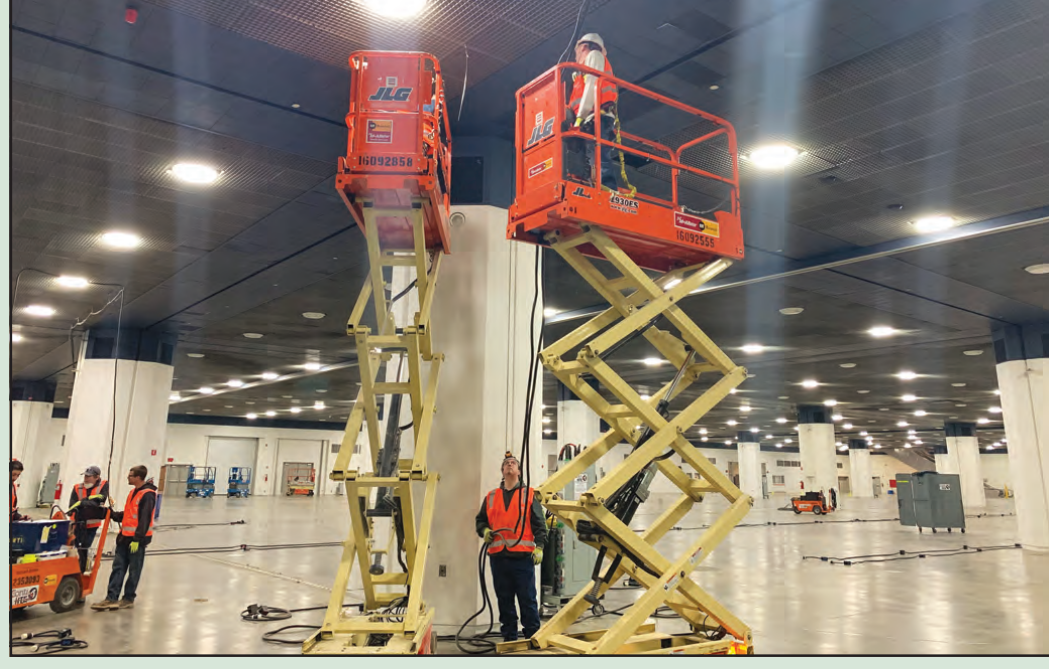
IBEW LOCAL 58 electricians help set up the TCF Center (formerly Cobo Hall) in Detroit as a field hospital to treat COVID patients.
