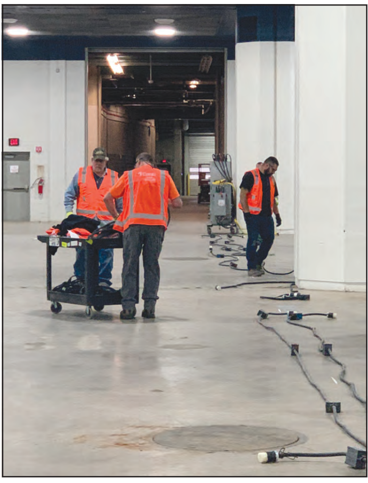
IBEW LOCAL 58 electricians employed by Conti help set up the TCF Center in Detroit as a COVID 19 medical center earlier this month.
