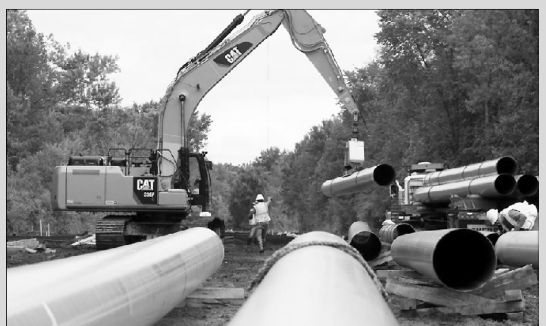
CONSUMERS ENERGY late last year completed construction of the 9-mile Saginaw Trail Pipeline, a natural gas line that dates to the 1940s. Photo credit: Consumers Energy
