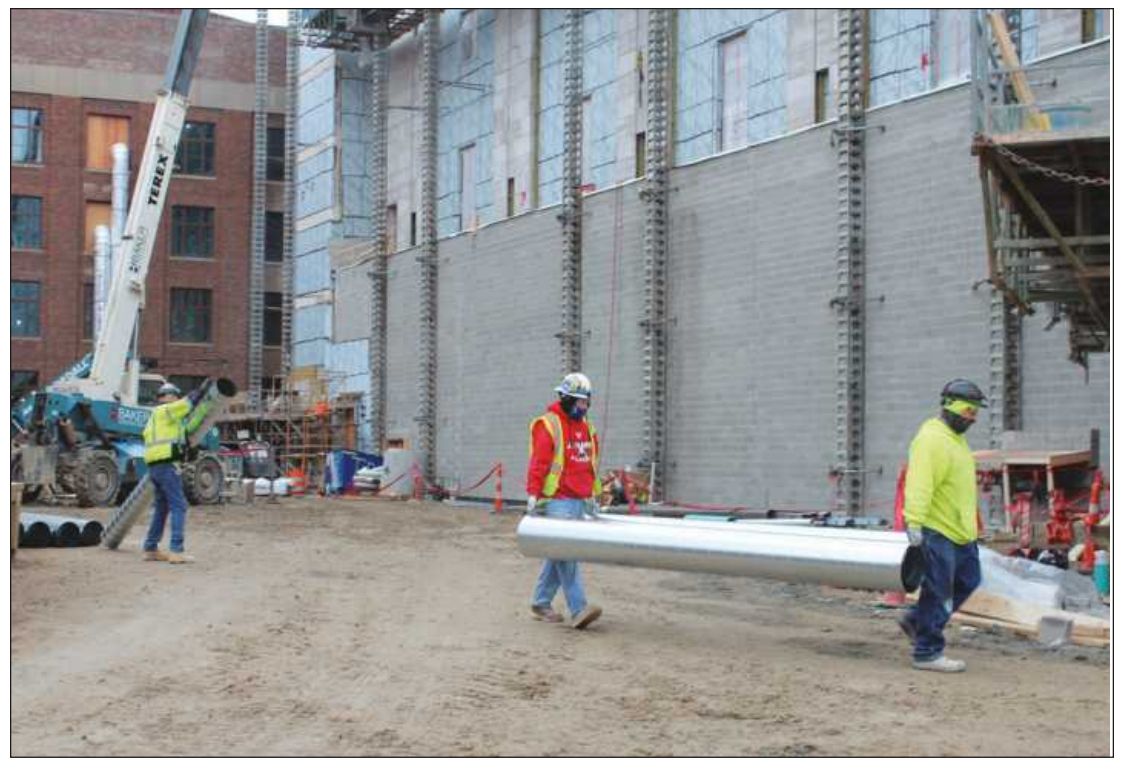
HEFTING DUCTWORK at the University of Michigan-Ann Arbor Central Classroom Building project are Mike Cassani, Bryant Stafford and Rik Watson of Sheet Metal Workers Local 80. They're employed by Applegate.
