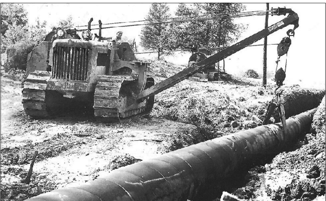
AN INTERNATIONAL-HARVESTER TD-24 from the late 1940s or early 1950s, fitted with a Superior side boom pipelayer, lowers a steel pipeline into a trench.
