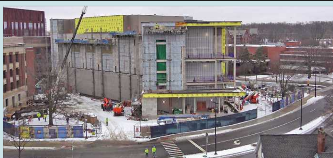
A NEW CENTRAL CLASSROOM Building is under construction on the University of Michigan campus at Geddes and Washtenaw Avenue. Barton Malow is managing construction of the $150 million project, which is being erected adjacent to the historic Ruthven Building, which is being renovated. Photo credit: U-M webcam
