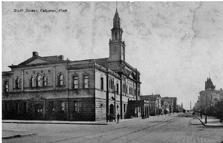
A 1910 POSTCARD view of the Calumet Theatre, surrounded by the town's brand new "granitoid" (concrete) pavement that was scored in a brick pattern to add aesthetics and improve traction for horses. The pavement installed here at Sixth and Elm streets has been repaved and covered over the years, but the oldest (1906) existing concrete still in place in Michigan can still be seen in a few blocks away.
