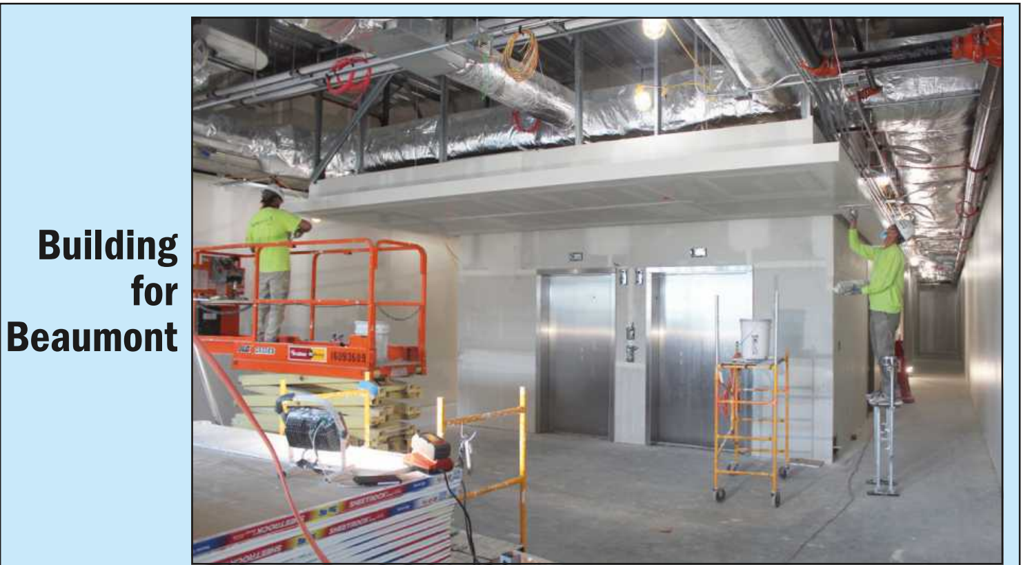
DRYWALLING AN ELEVATOR lobby at the Beaumont-Lenox Twp. Outpatient Campus are (l-r) Enrique Guillen and Guillermo Guillen of Michigan Painters District Council 1-M. They're employed by Denn-Co. Construction. The soon-to-open facility brings a new option for a full slate of health care services to northeast Macomb County in a three-story, 109,650-square-foot building erected near the intersection of I-94 and 26 Mile Rd. Roncelli is managing the project.
