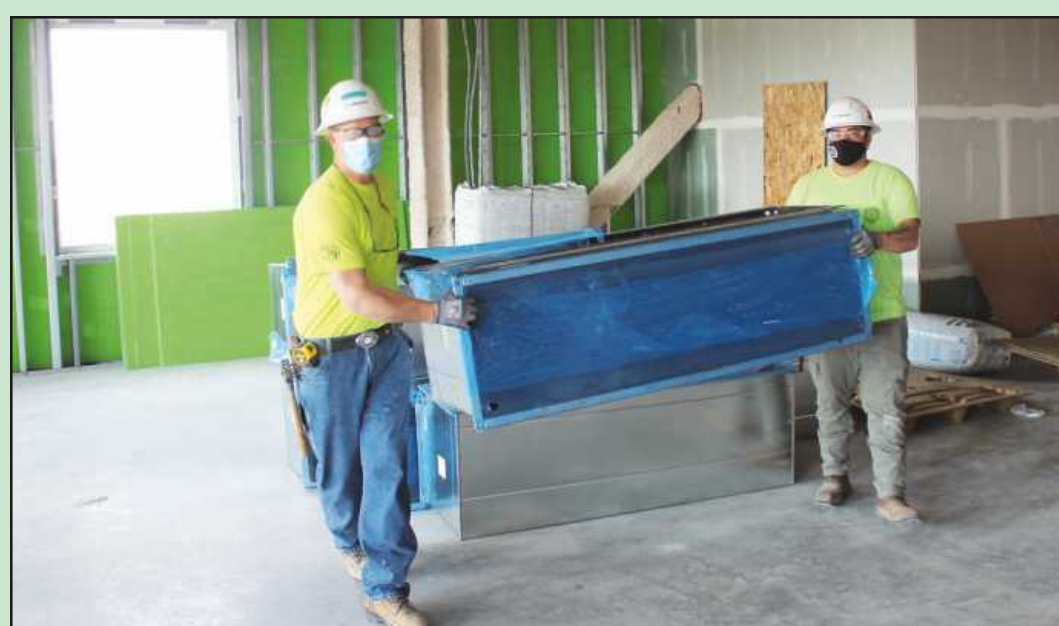
HEFTING A DUCT ELBOW SECTION across second-floor shell space at the Beaumont-Lenox Township facility are (l-r) foreman Chris Ratzel and Kody Gaffney of Sheet Metal Workers Local 80. They're employed by Limbach.
