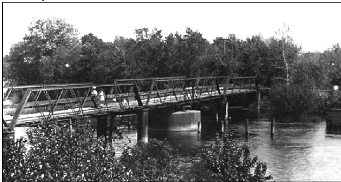
THE RICHMOND SWING BRIDGE in 1915. Historic Bridges noted that when the bridge was refurbished in 2005, it was dismantled "and the parts were repaired off-site before being returned to the site for reassembly. The bridge was restored in-kind and rivets were replaced with bolts, something that should be done automatically, however many states replace rivets with bolts, so this practice is worth mentioning." Photo credit: Fenville Memories
