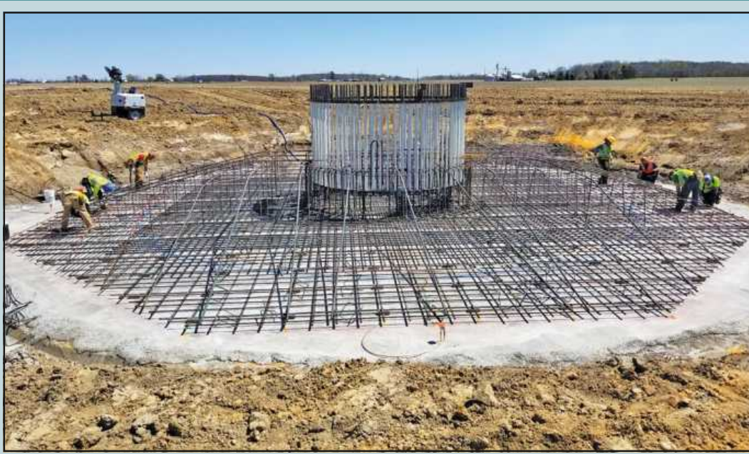
IRON WORKERS Local 25 rodbusters build the base of one of 60 wind turbines that will be erected this year for Consumers Energy's Gratiot Farms Wind Project in mid-Michigan's Gratiot County. They're employed by Barton Malow. Photo credit: Marc Crance
