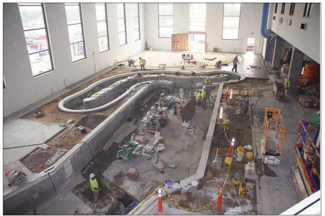
A MINI-WATER PARK is underconstruction on the ground floor of the expanded Island Resort Casino and hotel project.
