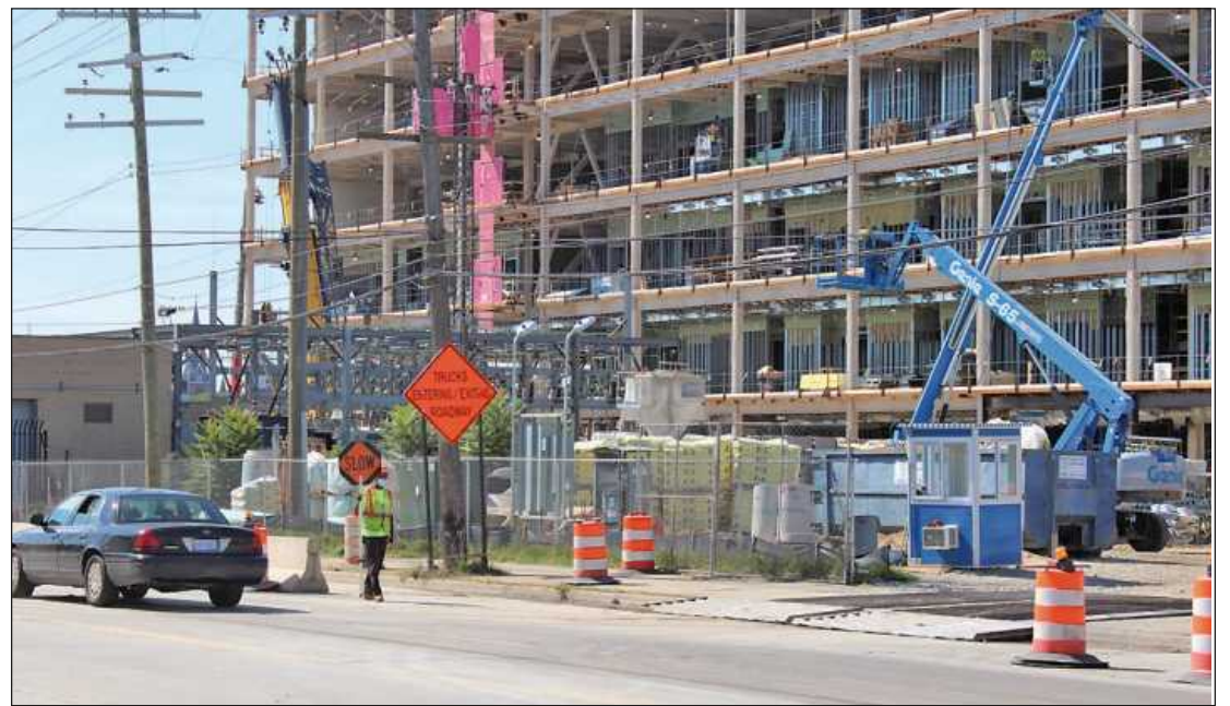
LABORER Reginald Miller of Local 1191 works traffic guidance on the Russell Street entrance to the Wayne County Detention Center, under construction in Detroit.
