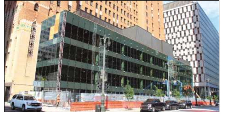
WHAT WILL BE the glass-encased Capital One Cafe, which seems like a "footstool" to the tall Guardian Building behind it.
