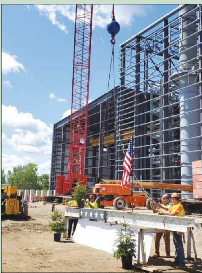
REDINGER STEEL iron workers set up the final beam for placement at the Delta Energy Park project. Photo credit: Marc Crance
