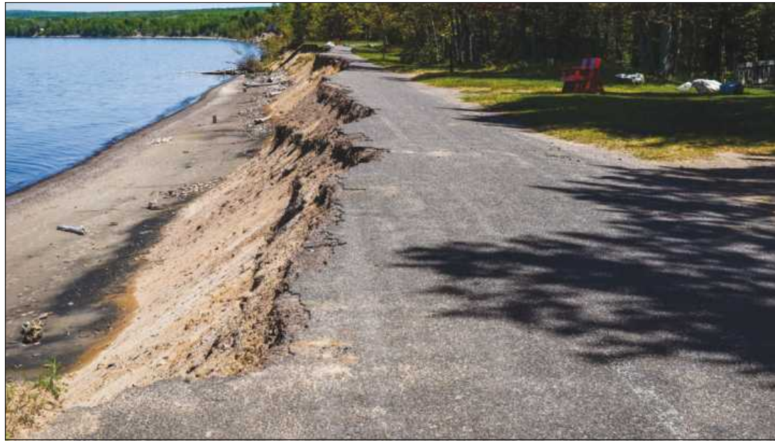
SIGNIFICANT EROSION plagued F.J. McLain State Park in Houghton County early in the Great Lakes high water levels crisis. Campsites, a park road and other features needed to be moved away from the shoreline.
