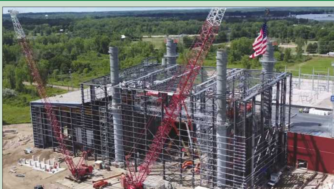
MORE THAN 1,300 tons of steel have been placed this year at the Lansing Board of Water and Light's Delta Energy Park, and the 250-megawatt power plant's structure was topped out on Aug. 6. Photo credit: Barton Malow video capture
