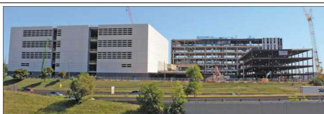
LOOKING EAST along I-75 is the new Wayne County Criminal Justice Center. Three of the five buildings at the site that are furthest along in construction are (l-r) the adult detention facility, the courthouse and the administration building.
