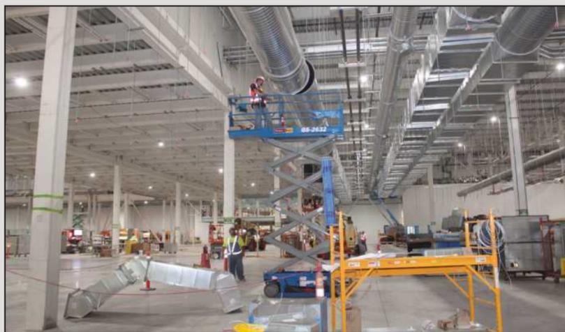
SETTING A 46-INCH DUCT at the Ultium Cells battery plant in Lansing are Josh Stone (on the lift) and James Medler. The Sheet Metal Workers Local 7 members are employed by Dee Cramer.
