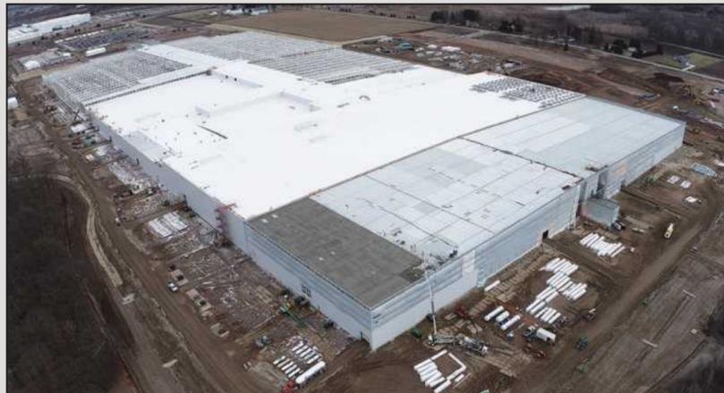
AT 2.8 MILLION SQUARE FEET, THE Ultium Cells plant under construction in Lansing along I-69 near I-96 is about as large as they come in Michigan. Currently it's mostly a shell inside, but in the coming months more than 1,000 building trades workers will be on site, installing hardware and systems to build electric-vehicle batteries. The project is a joint venture of LG Energy Solution and General Motors.
