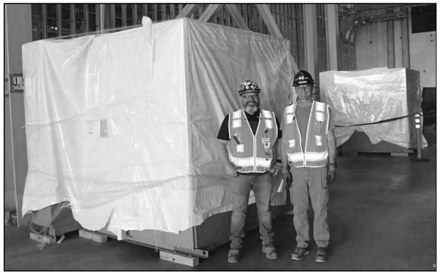
THE ROLE OF "Quality Control Inspector" is undertaken at the Ultium Cells battery plant by electrician Mike Arnot, right, of IBEW Local 665. Working for Superior Electric Great Lakes Co. and shown here with Superior Project Manager Ethan Eickelberg, Mike inspects hardware like the duplex switch under wraps next to them before it is wired into the Lansing plant.
