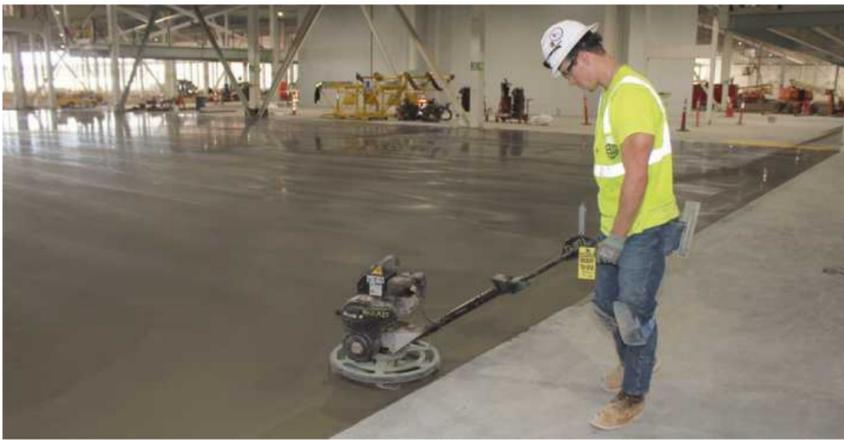
**SMOOTH OPERATOR:** Finishing part of the 2.8 million square-foot of floor at the Ultium Cells battery plant under construction in Lansing is Jeremy Pilch of Bricklayers and Allied Craftworkers Local 2. He's employed by Barton Malow.
