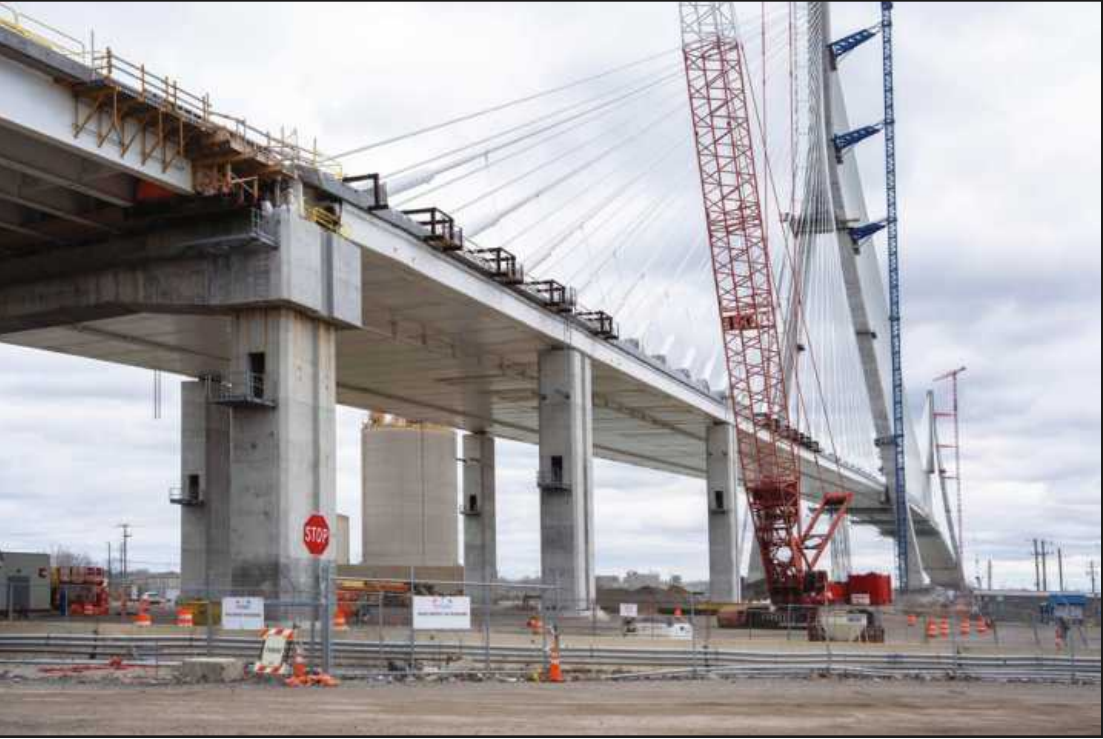
GORDIE HOWE BRIDGE designers employed an “unbalanced cantilever” system, with the back span of the road deck having been constructed first, supported by temporary falsework bents, before construction progressed on the main span over the Detroit River.
