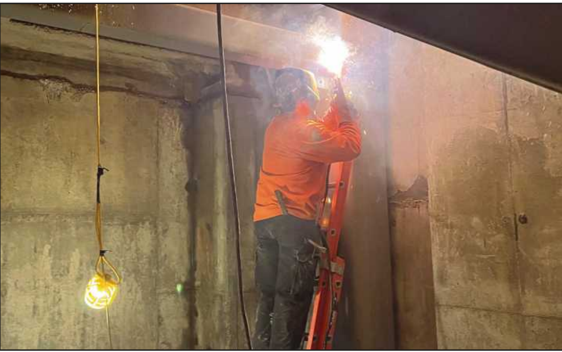
WELDING A STAIRWAY BRACE at Michigan State University’s Plant and Environmental Sciences Building in East Lansing is Scott Rumble of Iron Workers Local 25. He’s employed by Douglas Steel.
