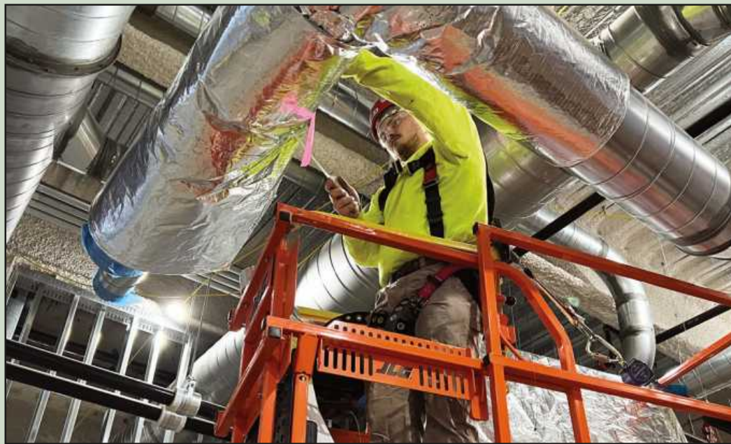
CUTTING DUCT INSULATION on the first floor of the Plant and Environmental Science Building on the MSU campus is Jacob McCormick of Heat and Frost Insulators Local 47. He's employed by Mechanical and Industrial Insulation.
