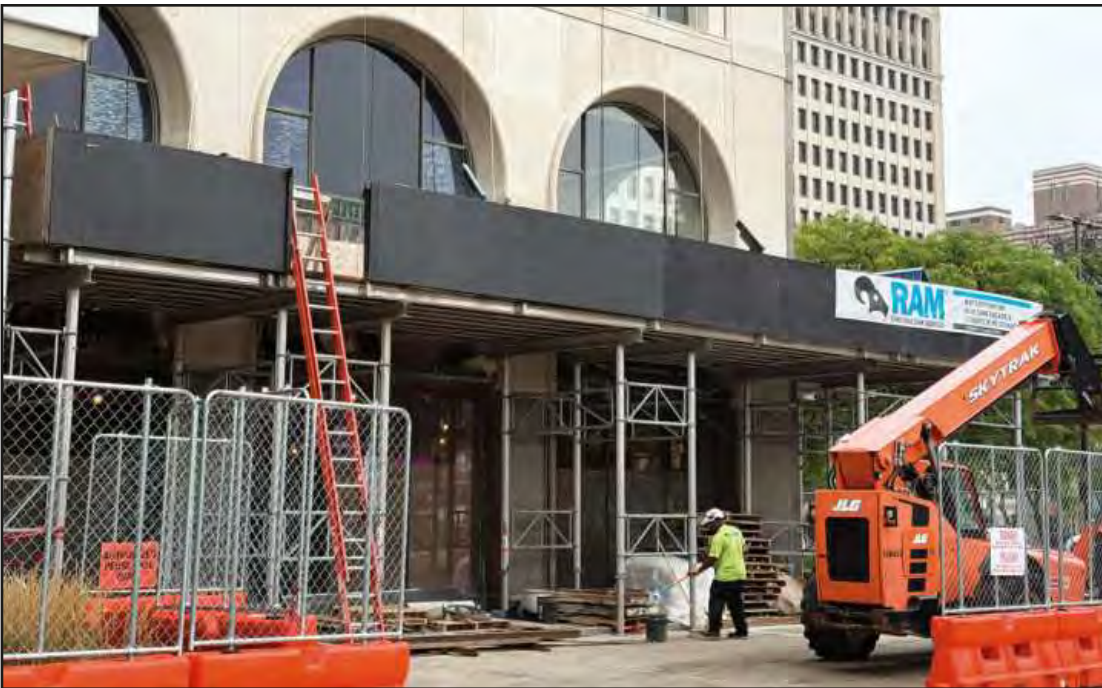
TIDYING UP on the west side of the Fisher Building in Detroit is Anthony Dyson of Laborers Local 1191. He’s employed by RAM Construction Services.
