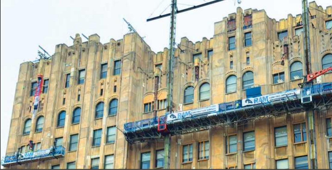
SCAFFOLDING SUPPORTS RAM Construction Services masons working on the Fisher Building in Detroit.
