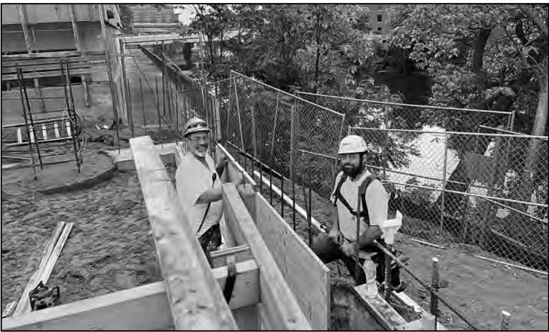
PLACING A CONCRETE wall form at the Tower on Grand project in Lansing are carpenters Bill Kogagen (Local 687) and Jared Bolan (Local 1004). The Michigan Regional Carpenters Council members are employed by Baker Construction,
