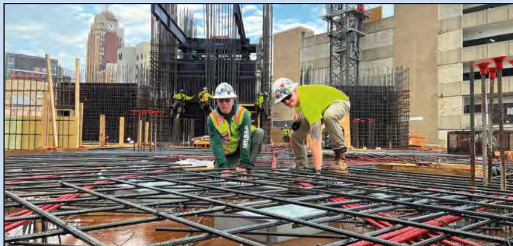
WORKING BETWEEN THE re-rod maze setting electrical non-metallic tubing at the Tower on Grand site in Lansing are (l-r) IBEW Local 665 electricians Matt Hunter and Sean Archey. They're employed by Superior Electric Great Lakes Co.
