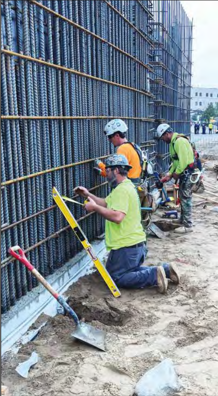
MAKING PREPARATIONS to set wall panels outside the field of re-bar at the Tower on Grand project in Lansing are carpenters James Klingenberg, Kenny Crouch and Jason Smith. The Michigan Regional Carpenters Council Local 1004 members are employed by Baker Construction.
