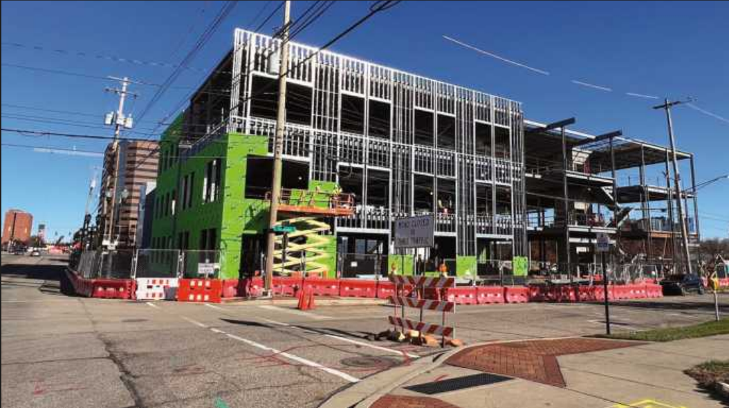
GOING UP AT THE CORNER of Lenawee Street and Grand Avenue in Lansing is what will be a modern, long-awaited city hall. Construction of the 65,000 square-foot building is being managed by Clark Construction.
