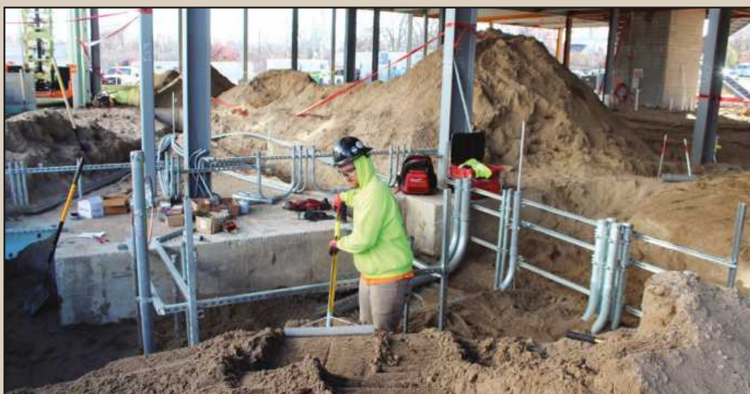
AT LANSING’S NEW CITY HALL project, earlier this month electricians on the ground floor were in their “landscaping mode,” moving around the sandy soil to cover the conduit they installed. At work here doing some backfilling is Gavin Grinstern of IBEW Local 665. He’s employed by Centennial Electric.
