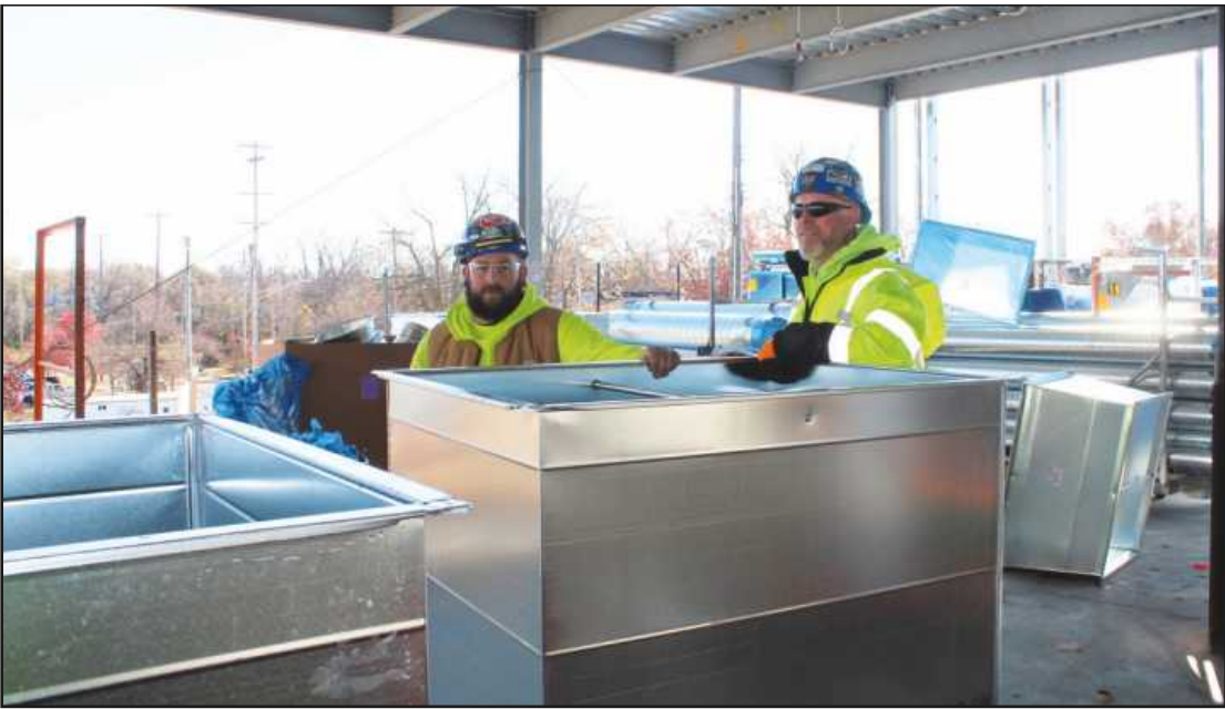
SUPPLY AIR DUCTS at the new Lansing City Hall project are handled by Bruce Westen and Kirk Densmore of Sheet Metal Workers Local 7. They’re employed by Dee Cramer.
