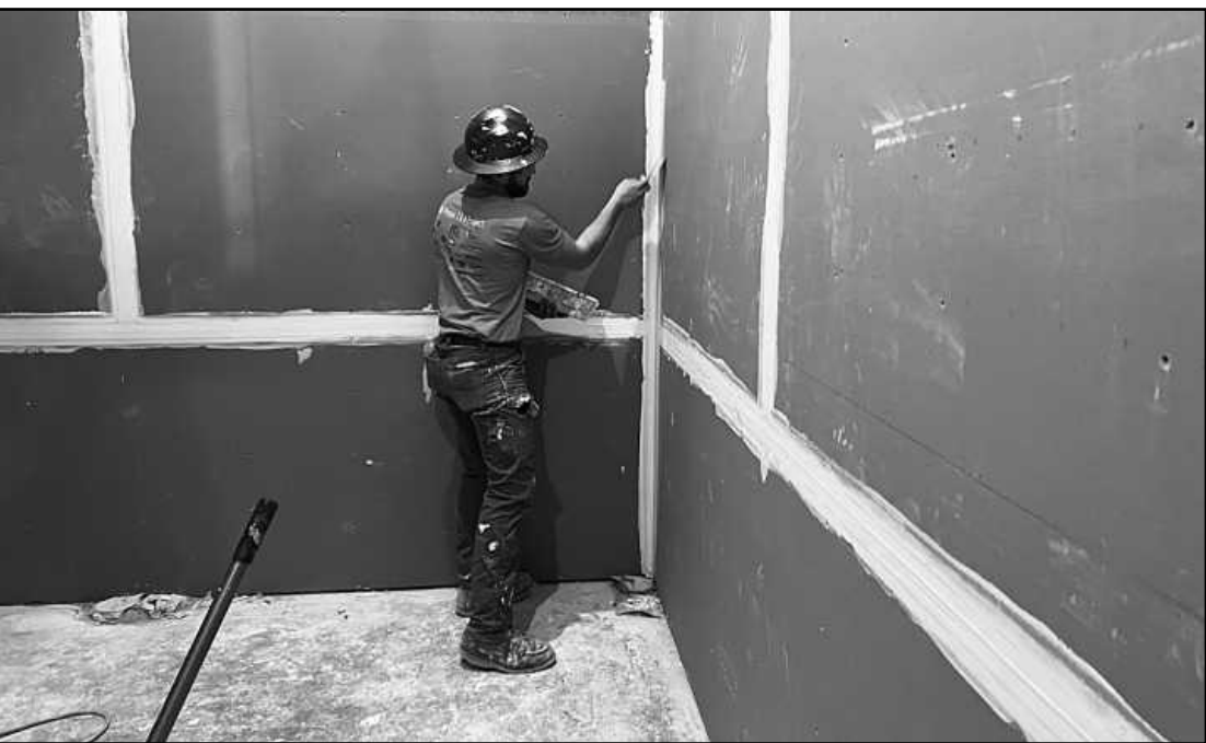
MUDDING DRYWALL in an electrical room at the MSU Plant and Science Building in East Lansing is Tayler Wilkins of the Michigan Painters District Council Local 845. He's employed by Integrity Interiors.
