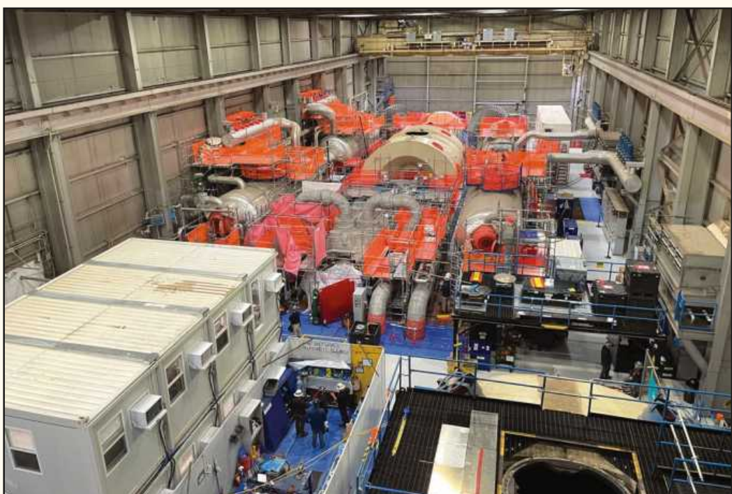
THE TURBINE FLOOR at the Palisades Nuclear Power Plant last year. The Westinghouse turbine has been disassembled, inspected, and repaired where needed, and will be a key piece of infrastructure when the restored plant starts to create electricity this year.
