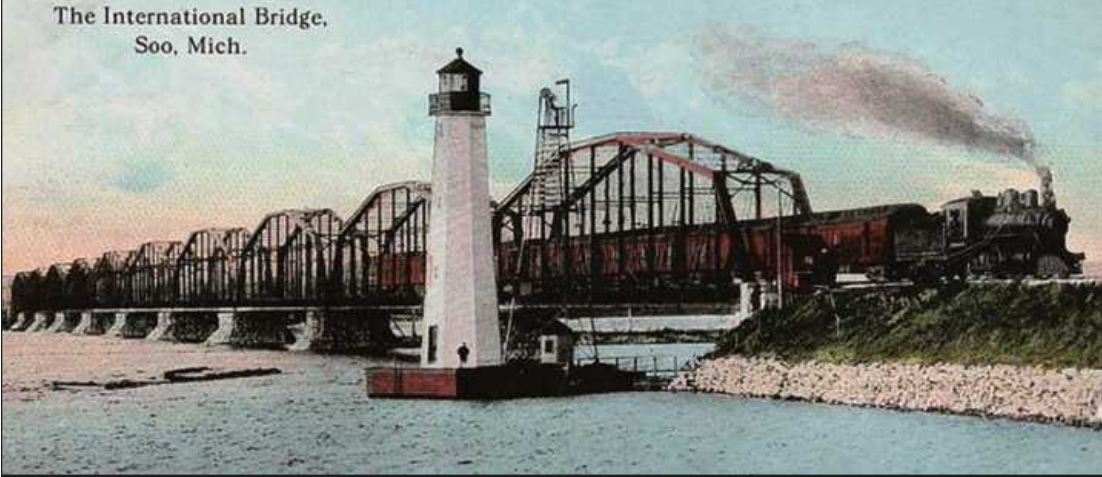
A SERIES OF NINE “Camelback” steel trusses, built in 1887, comprise an original section of the Sault Ste. Marie International Railroad Bridge. Here is a 1914 postcard, showing the camelback through-trusses, each 239 feet long, resting on finished ashlar piers (squared building stones) anchored in the bedrock of the river. One of these trusses was removed to enable construction of the bascule bridge section. Various other elements of the bridge have been replaced over the years.
