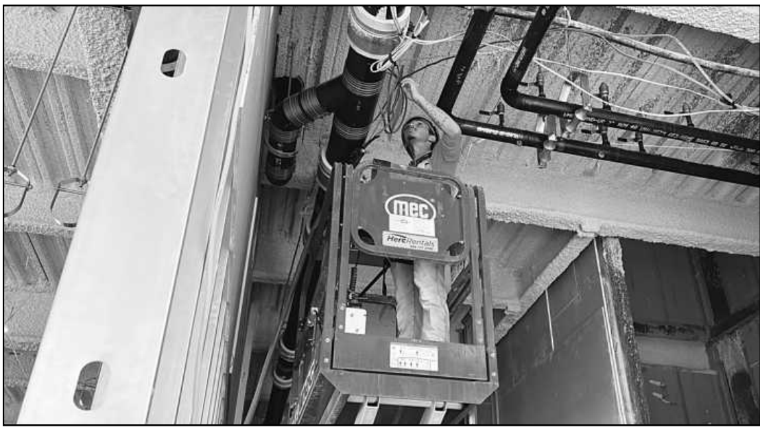
SETTING A STORM DRAIN at the Michigan State University's Plant and Environmental Science Building in East Lansing is Gavin Hinds of Plumbers and Pipe Fitters Local 333. He's employed by John E. Green.
