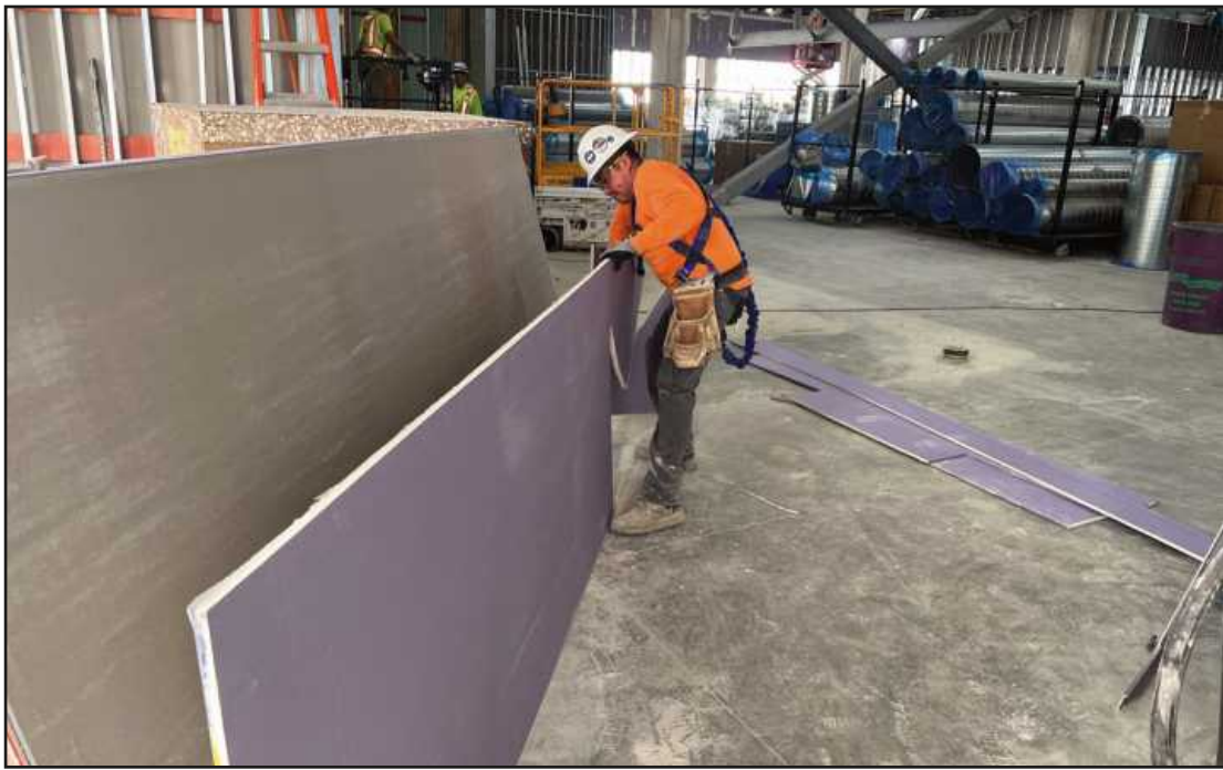
CUTTING DRYWALL at the MSU Plant and Environmental Sciences building in East Lansing is Mario Alberto Zayas of Michigan Regional Carpenters Council Local 525. He’s employed by Integrity Interiors.
