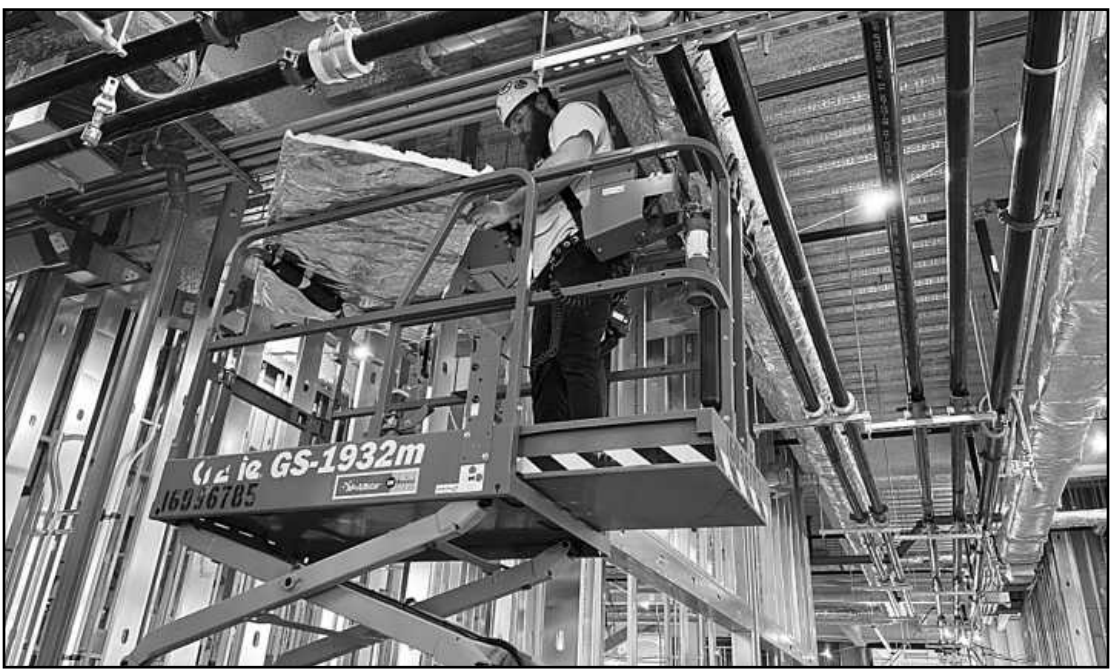
HEAT AND FROST INSULATOR Brad Schmitzer of Local 47 cuts a piece of insulation while working at the MSU Plant and Environmental Science Building in East Lansing. He's employed by Mechanical and Industrial Insulation.
