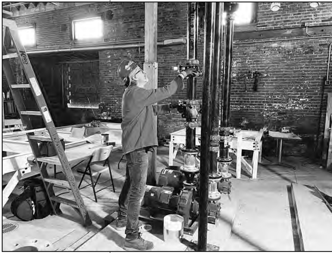
SETTING UP THE HARDWARE for the HVAC heating pump in the mechanical room at the Belle Isle Aquarium in Detroit is Justin Peters of Pipe Fitters Local 636. He's employed by Watson Brothers.
