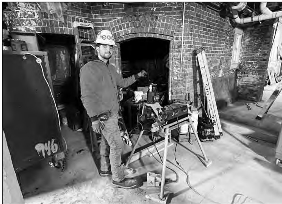
GROOVING A 4-INCH Schedule 40 heating and cooling pipe at the Belle Isle Aquarium project in Detroit is Mason Vandekerckhove of Pipe Fitters 636. He's employed by Watson Brothers.
