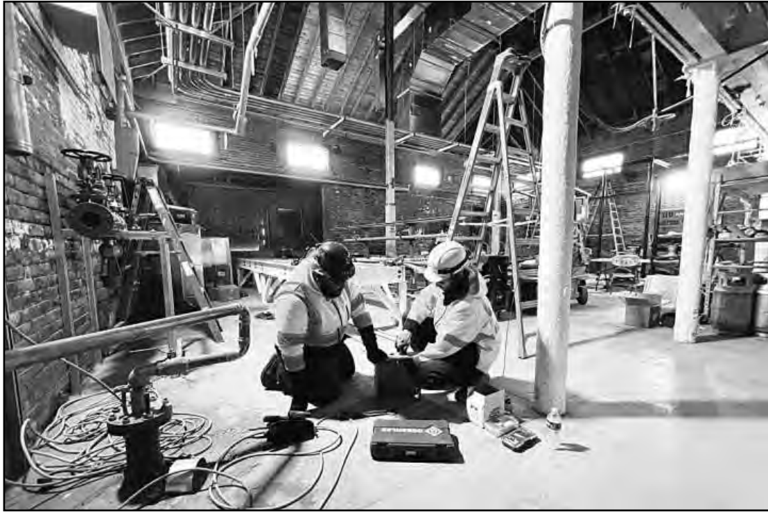
SETTING UP A BOX to terminate conduit at the Belle Isle Aquarium project in Detroit are electricians Chase Dockery and Cameron Sellers. The IBEW Local 58 members are employed by Control Solutions.
