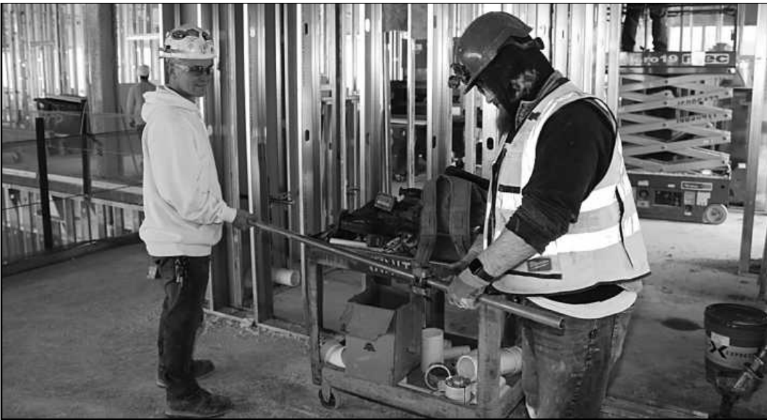
CUTTING DOMESTIC water pipe at the Northville Twp. psychiatric hospital project are (l-r) Kyle Flint and Mike Wendell of Plumbers Local 98. They’re employed by Conti.
