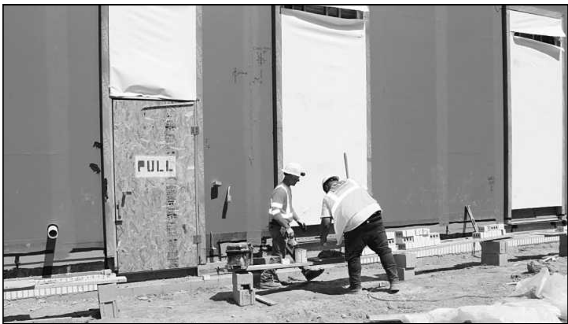
STARTING WORK on setting a brick wall course at the Northville Twp. psychiatric hospital site are mason foreman Joe Kalthorn of Bricklayers and Allied Craftworkers Local 2 and Brandin Stout of Laborers Local 1191. They’re employed by Leidal and Hart.
