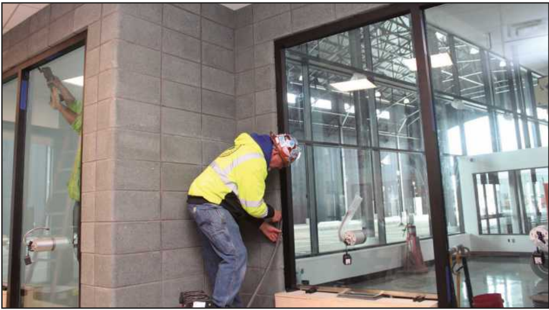
SETTING BACKER ROD while setting an interior ticket window at the Jason Hargrove Transit Center is the aptly named Ethan Glass of Glaziers and Glassworkers Local 357. He's employed by Peterson Glass.
