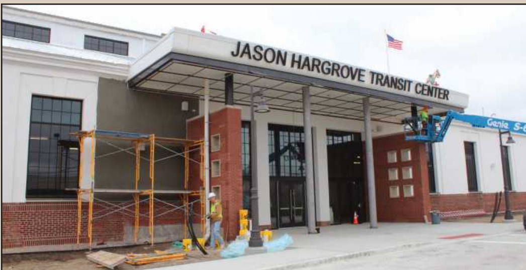
TWO TRADESMEN ARE shown here putting final touches on the main entrance to the Jason Hargrove Transite Center in Detroit. At left is plasterer Scott Helig of Plasterers and Cement Masons Local 514, who is applying stucco to the exterior walls. He's employed by Russell Plastering. On the left is Bill Heety of Carpenters Local 687, employed by Diversified Metal Fabricators.
