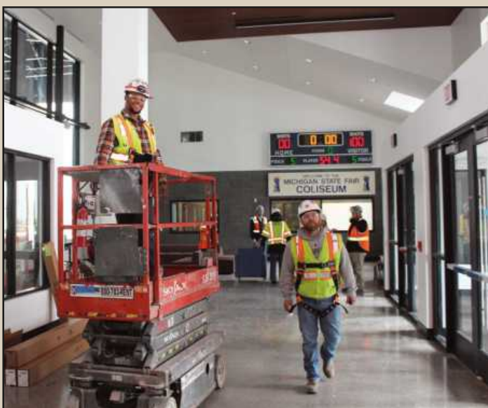
AT WORK IN THE LOBBY of the new transit center in Detroit are electricians Jake Brock (on the left) and Rob Golenbiewski. The IBEW Local 58 members are employed by Detroit Power Systems. Behind them on the wall, the scoreboard and sign from the demolished Michigan State Fair Coliseum were incorporated into the new lobby.
