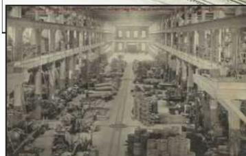
THE SHEFFIELD CAR Co.'s seven-acre campus is shown above in 1895. At left, the assembly plant in 1910 is shown making railroad inspection handcars and stand pipes used to rewater steam engines. In 1895 the campus was powered by both hydro and utility-provided electricity, lighting 150 incandescent bulbs. The campus included a foundry, designing offices, woodworking, paint, erecting buildings, and a power plant. At its peak, 1,500 were employed there.
