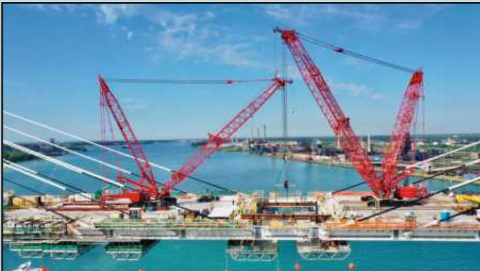
A FINAL STEP in the Gordie Howe Bridge’s construction over the Detroit River was the placement of a temporary connection using temporary steel braces. Congratulations on a safe, well-done job to the entire Bridging North America workforce.
