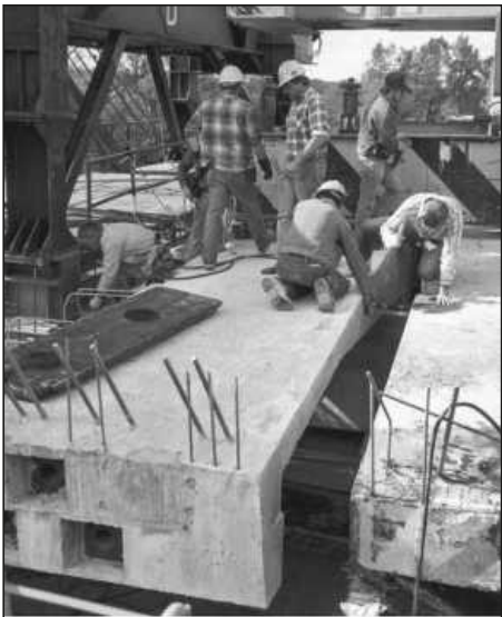
PLACEMENT OF A CONCRETE section is shown on the Zilwaukee Bridge.
