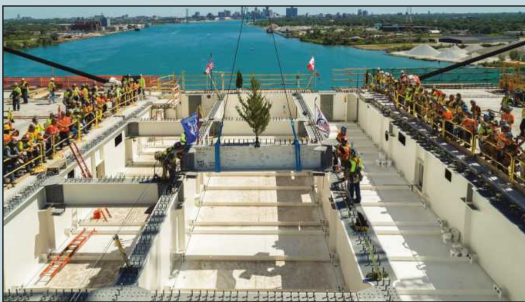
UNION IRON WORKERS from the Detroit and Windsor side of the Gordie Howe Bridge meet in the middle of the span on June 14, marking the span’s final connection with the traditional fir tree and topping out ceremony.
