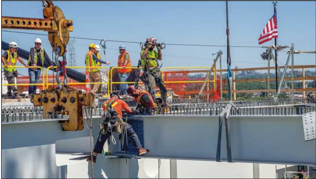
IRON WORKERS set a piece of steel to support the final connection of the Gordie Howe Bridge this month.
