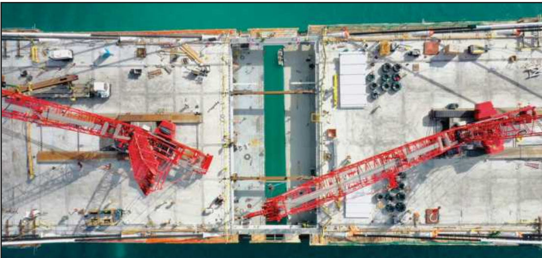
A GREAT LAKES bulk freighter slides under the newly connected Gordie Howe Bridge. Below, the bridge awaits placmenet of the its final deck segment.
