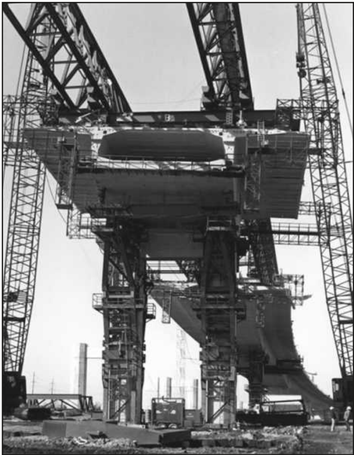
A CUTAWAY of the Zilwaukee's segmented box girder design during construction.
