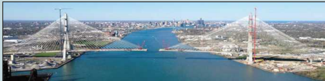
TWIN 722-FOOT-TALL towers support the .53-mile main span of the Gordie Howe Bridge between Detroit and Windsor, making it the longest main span of any cable-stayed bridge in North America. The total length of the bridge is 1.5 miles. This photo was taken last month, when the gap between the bridge decks was about 85 feet.
