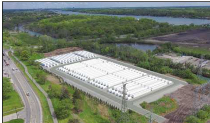
ON THE SITE of the soon-to-be demolished Trenton Channel power plant, DTE Energy is planning the construction of a 220-megawatt energy storage center – the largest in the Great Lakes Region. This is a DTE Energy rendering of the project.
