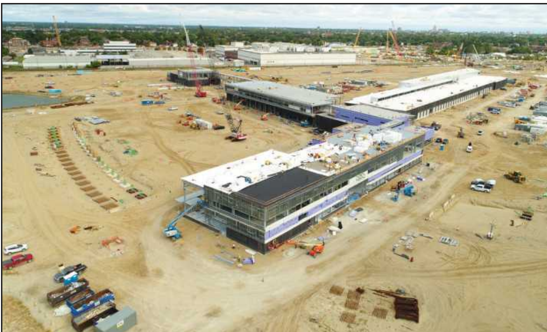
THE U.S. Point of Entry in Southwest Detroit connected to the Gordie Howe Bridge consists of a massive 167-acre site cleared of all buildings. Being erected as part of the project are 13 buildings, which will comprise one of the largest border crossings in the U.S.
