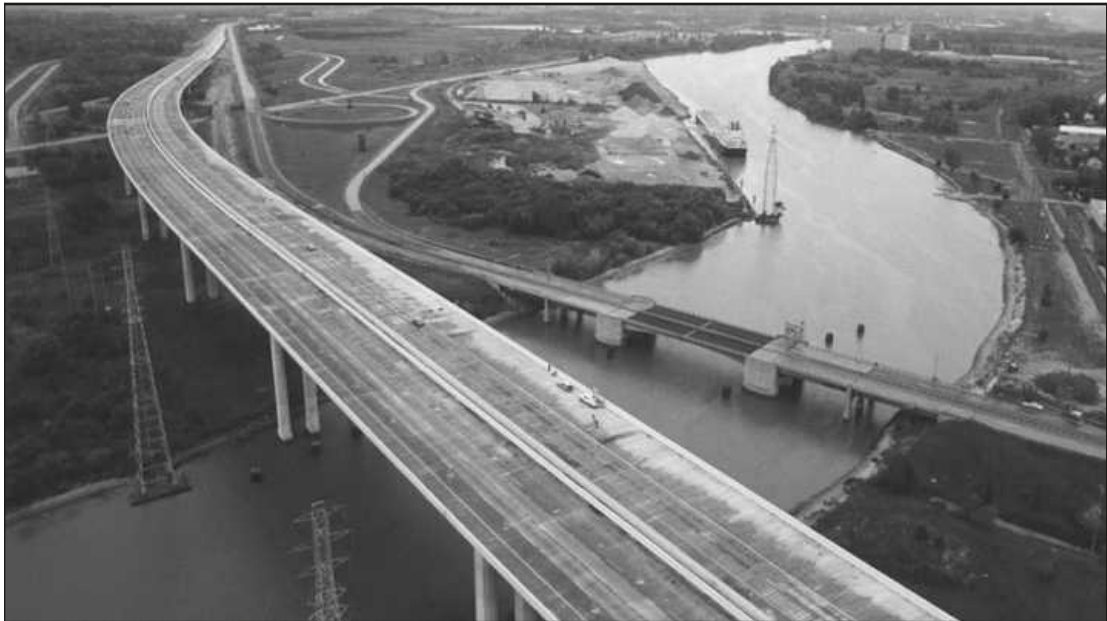
THE EIGHT-LANE ZILWAUKEE BRIDGE that carries I-75 traffic 125 feet over the Saginaw River hasn't won any architectural design contests, but it has been a vast improvement for motorists, compared to the four-lane drawbridge next door that it replaced in 1988. The drawbridge was later demolished.
