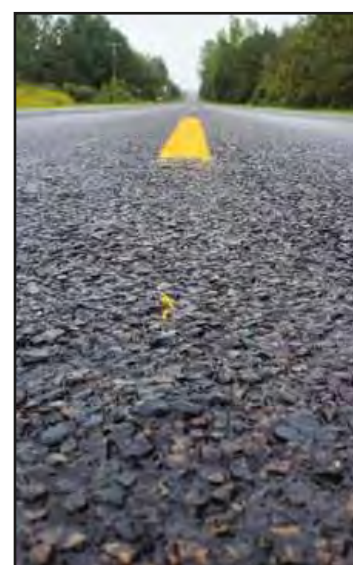
A RUBBER-MODIFIED chipseal application is shown on Saganing Rd. in Bay County.
