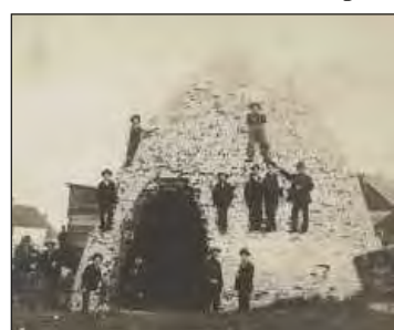
A BEEHIVE charcoal kiln at Carp River kiln off of M-28 in the Upper Peninsula, like the kind that fed the Elk Rapids plant.
