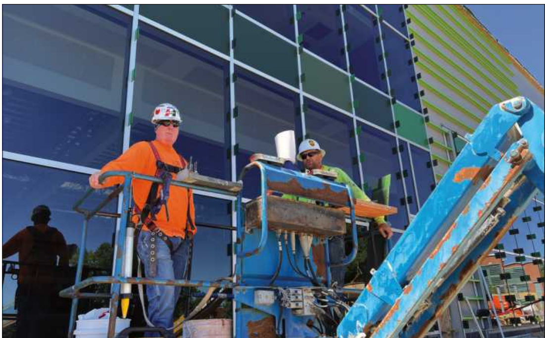
INSTALLING SUN SHADE fixtures on the exterior of the Michigan State University Multicultural Center in East Lansing are Glaziers and Glassworkers Local 826 members Erik Mitchell and Troy Hill. They are employed by Glazing Solutions.
