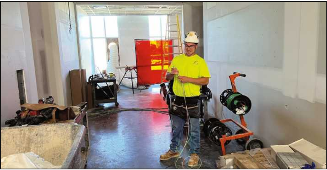
SETTING UP A LENGTH of No. 12 lighting wire at the MSU Multicultural project in East Lansing is electrician Jacob Edgman of IBEW Local 665. He’s employed by Centennial Electric.
