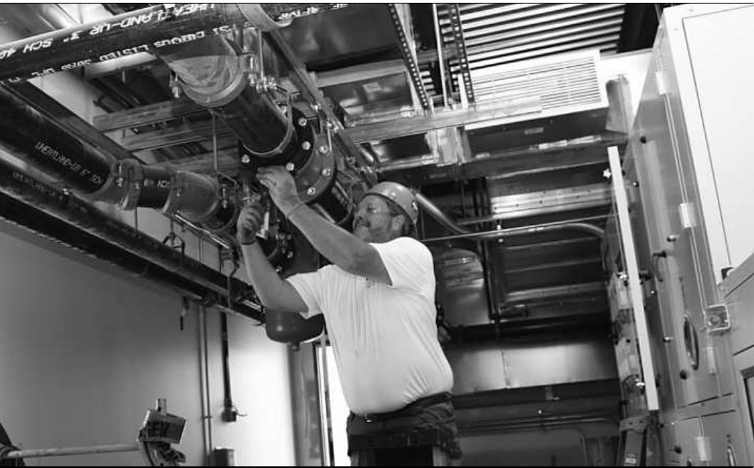
SETTING BOLTS ON a six-inch condensed water pipe at the Michigan State University Multicultural Center project is Blain Lysher of Plumbers and Pipe Fitters Local 333. He's employed by Myers Plumbing and Heating.
