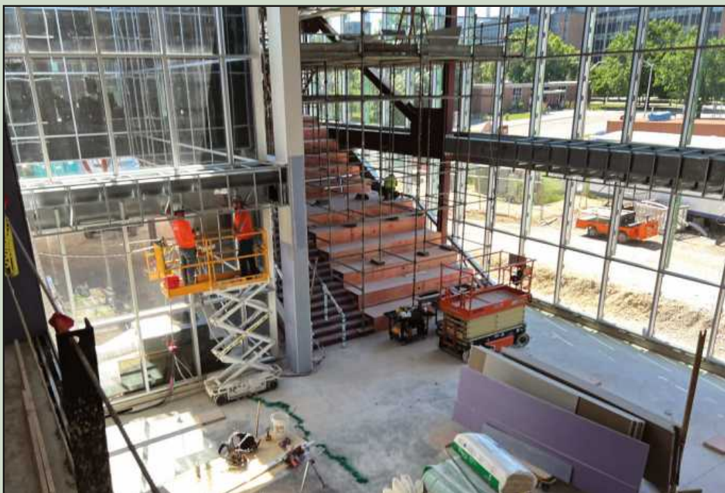
SETTING RADIANT thin tube piping in the two-story "living room" of the Multicultural Center on the Michigan State University campus in East Lansing are Josh Wilk and Dusty Seavolt of Plumbers and Pipe Fitters Local 333. They're employed by Myers Plumbing and Heating.
