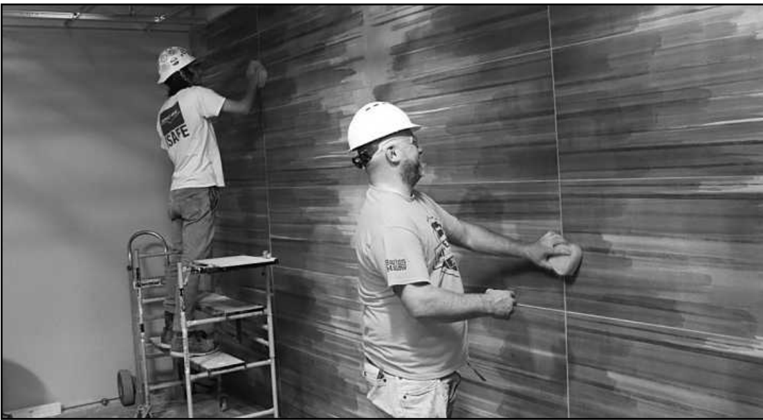
SPONGING A WALL in the ablation room at the Michigan State University Multicultural Center project are Bricklayers and Allied Craftworkers Local 2 masons Vincent Cecora and Bob Voss. They're employed by Integrity Interiors.
