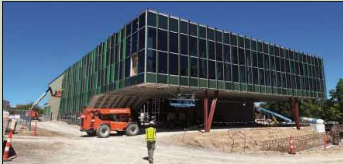
MODERN ELEMENTS – with a cantilevered front and walls of green glass – help shape the 34,000-square-foot Multicultural Center at Michigan State University. The team of Clark Construction /White Construction are managing the project.
