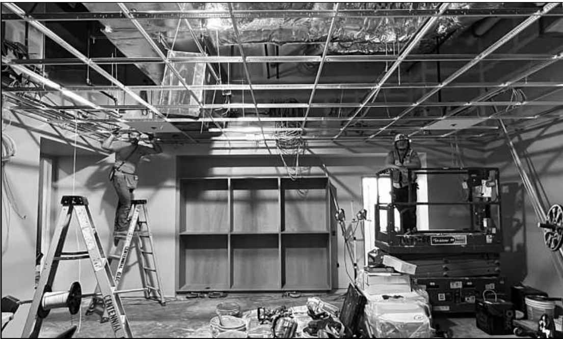
APPRENTICE ELECTRICIANS Hunter Hohman and Brendan Young of IBEW Local 665 were pulling wire in the Group Reflection Room at the Michigan State University Multicultural Center in East Lansing when we asked them to come down under the ceiling grid to have their photo taken. They're employed by Centennial Electric.
