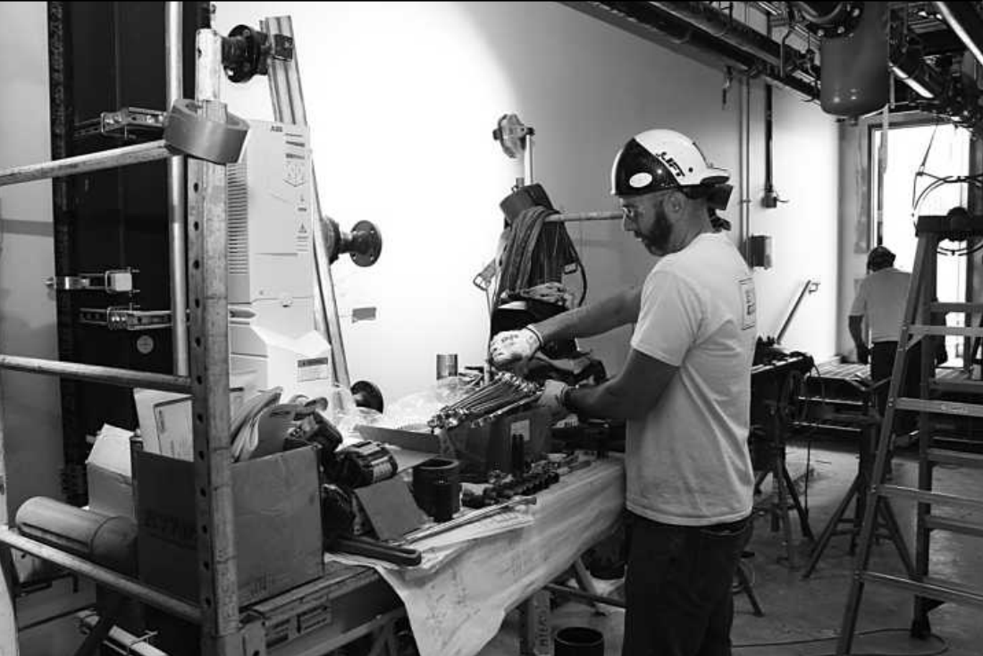
SETTING UP TOOLS on a workbench at the MSU Multicultural Center project at Michigan State University is Sean Castillo of Plumbers and Pipe Fitters Local 333. He's employed by Myers Plumbing and Heating.
