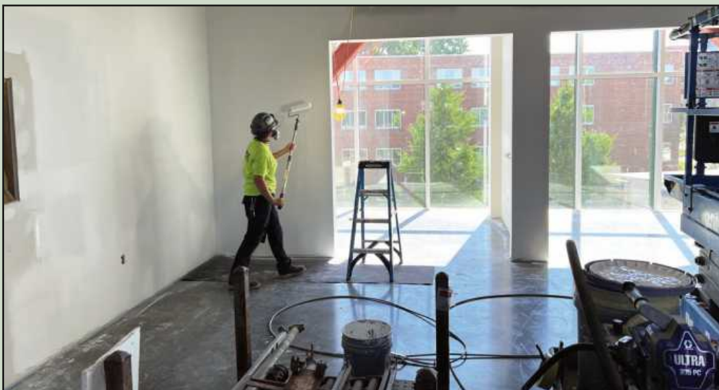
PAINTING A WALL in the "hoteling" (temporary office) area at the MSU Multicultural Center project in East Lansing is Christina Pettigrew of Painters Local 1052. She's employed by Murray Painting.
