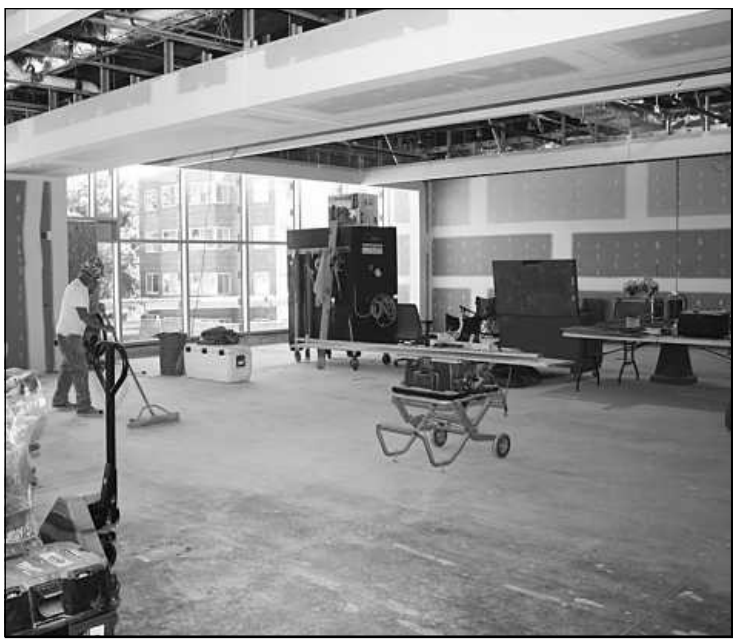
TIDYING UP what will be the multipurpose room at the MSU Multicultural Center project in East Lansing is laborer Darren Dayton of Local 499. He's employed by Christman.
