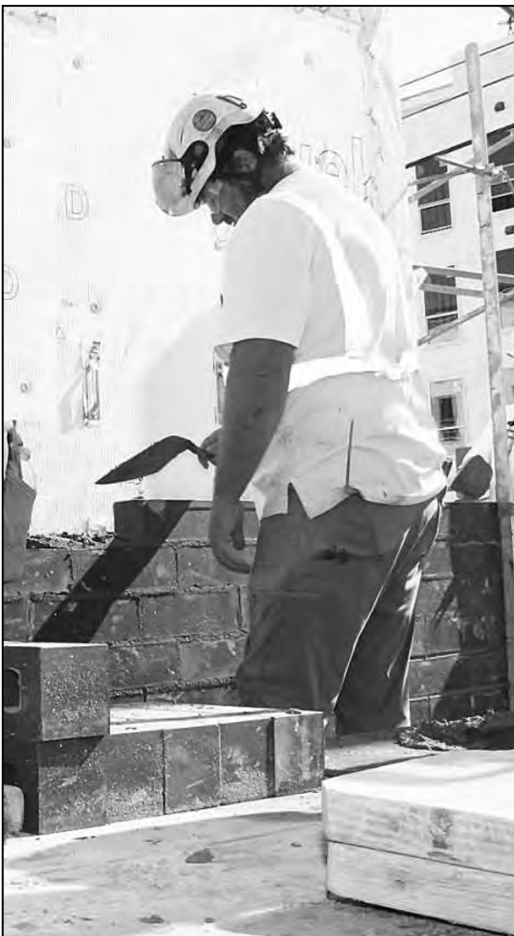
LAYING A BRICK WALL at the Northern Michigan University Presque Isle apartment site is Pete Johnson of Bricklayers and Allied Craftworkers Local 2. He's employed by Boettcher Masonry.
