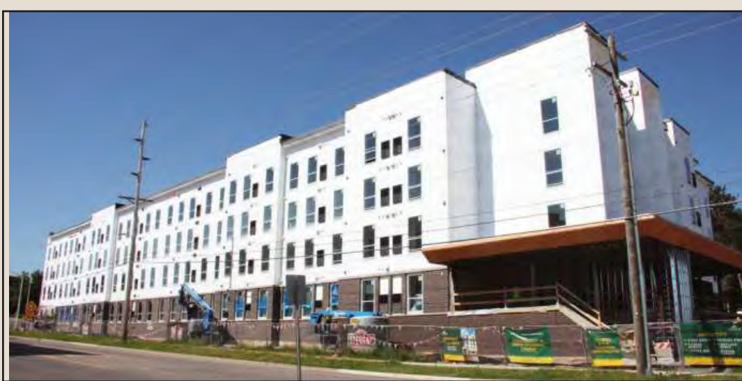
CONSTRUCTION WAS PROCEEDING on schedule last month at one of the two Northern Michigan University residence halls along Presque Isle Avenue. Construction of the $55 million project has been led by Stevens Construction, and is expected to wrap up in time for the 2027 fall academic semester.
