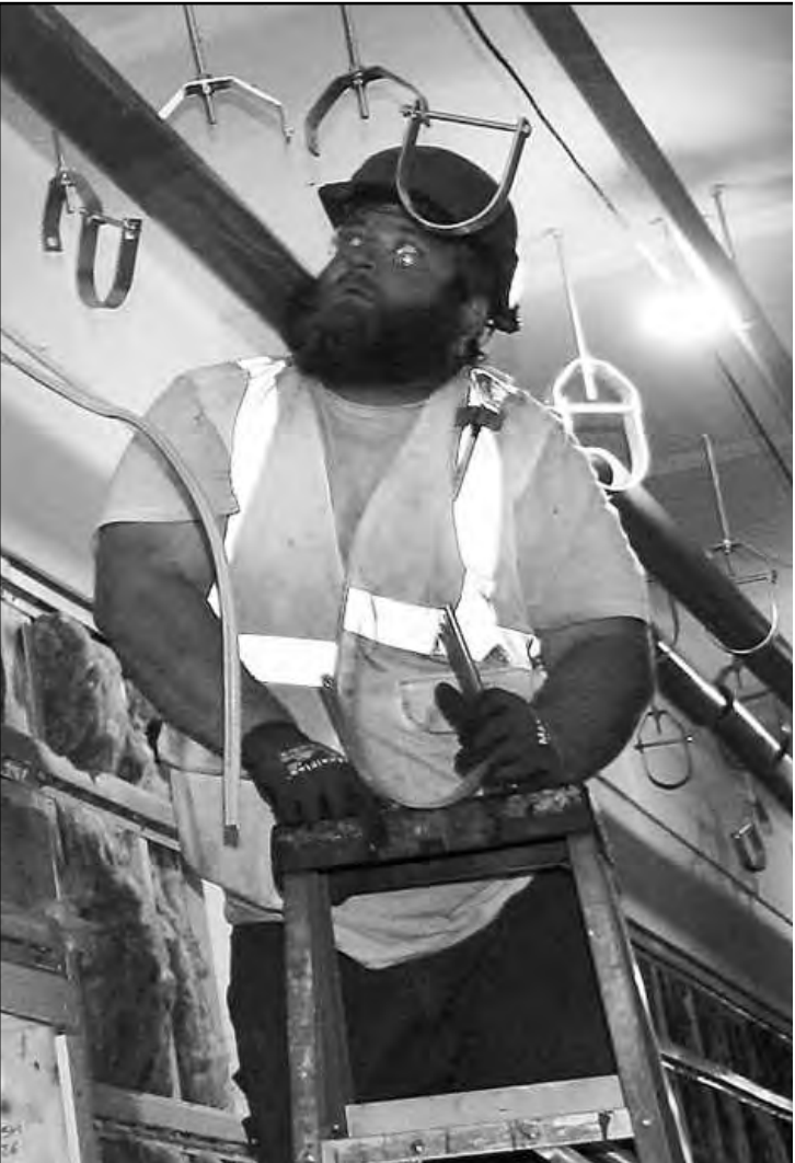
SETTING PIPE HANGERS in a hallway at the Northern Michigan University Presque Isle residence halls project is Dustin Reinhart of Plumbers and Pipe Fitters Local 111. He’s employed by Dressler Mechanical.
