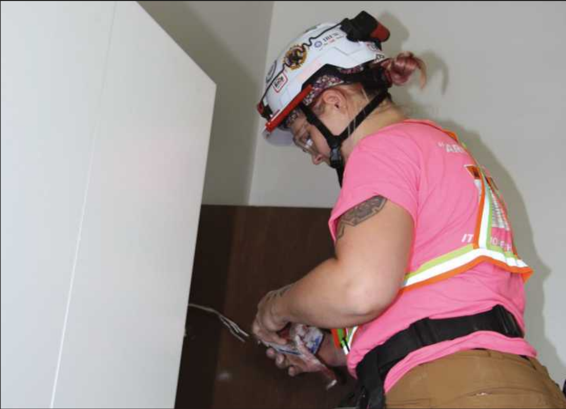
AT WORK ON AN ELECTRICAL box at the NMU Presque Isle apartments project in Marquette is Freya Wiser of IBEW Local 906. She’s employed by Pieper Electric.
