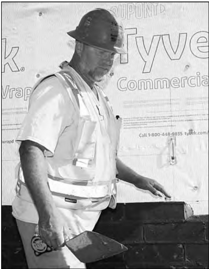
LAYING A BRICK WALL at the Northern Michigan University Presque Isle apartment site is David Saari of Bricklayers and Allied Craftworkers Local 2. He's employed by Boettcher Masonry.
