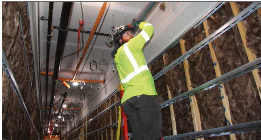
INSTALLING A PIPE in a hallway at the Northern Michigan University Presque Isle residence halls project is Robert Glover of Plumbers and Pipe Fitters Local 111. He's employed by Dressler Mechanical.
