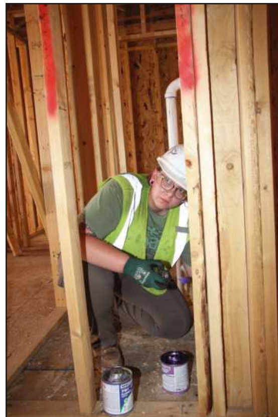
GLUING PVC pipe at the NMU Presque Isle apartments project is Emma Heinz of Plumbers and Pipe Fitters Local 111. She's employed by Dressler Mechanical.
