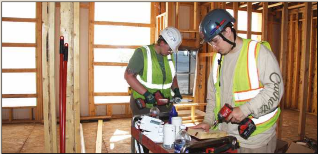
ASSEMBLING FIXTURES for installation at the Northern Michigan University Presque Isle apartments project in Marquette are Emma Heinz and Landon Reichel of Plumbers and Pipe Fitters Local 111. They're employed by Dressler Mechanical.
