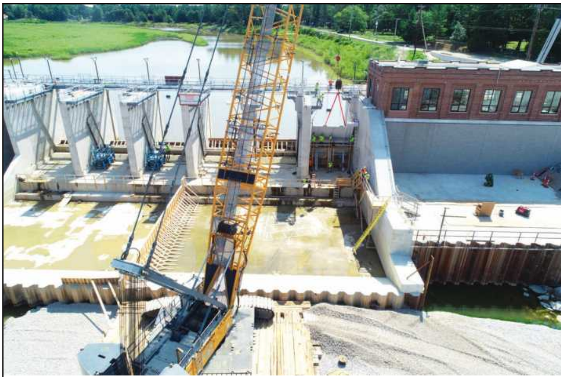
THE REBUILT SANFORD Dam is shown with the setting of its first crest gate in August, a milestone announced early last month by Spence Brothers. The failed earthen dam collapsed after heavy rains in 2020; the replacement dam involves the placement of thousands of yards of new concrete.
