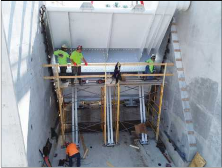
A CREST GATE on the Sanford Dam is installed by building trades workers.
