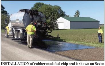
Mile Road in Bay County. The use of rubberized asphalt-based products on road work is accelerating in Michigan.
