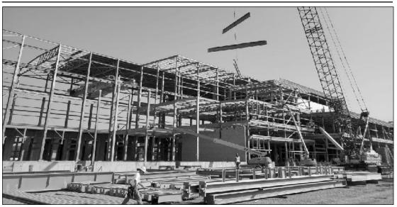
IRON WORK AT the Graphics Packaging plant in Kalamazoo proceeds in September. Doing the structural iron work are Local 25 members employed by Barton Malow erectors. The \$600 million plant at 1500 N. Pitcher Street will have the ability to produce 500,000 tons of recycled paperboard per year. It will house a coated recycled board (CRB) machine, which the company says "is designed to be the largest and lowest cost producer of CRB in North America." Photo credit: Marc Crance
