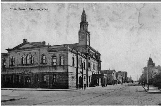
A 1910 POSTCARD view of the Calumet Theatre, surrounded by the town's brand new "granitoid' (concrete) pavement that was scored in a brick pattern to add aesthetics and improve traction for horses. The payement installed here at Sixth and Elm streets has been repayed and covered over the years, but the oldest (1906) existant concrete still in place in Michigan can still be see a few blocks Photo credit: Detroit Public Library
