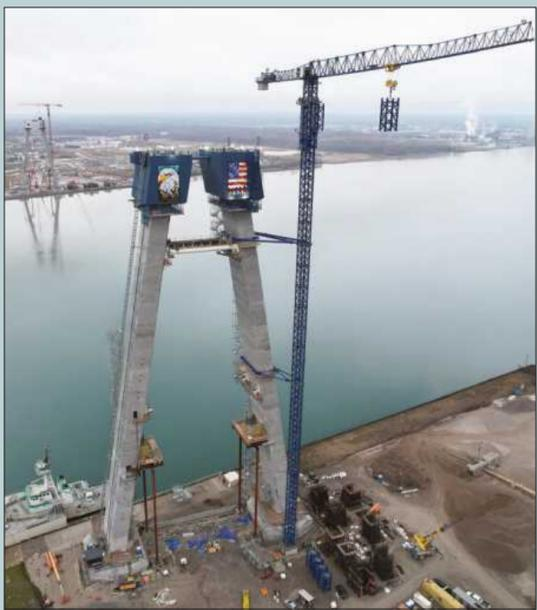
**WITHIN THE FORMS** at the top of the legs, according to *Construction Connect*, concrete is poured through rebar, with a total of about 130 cubic yards for a typical "lift" or segment. The forms then "climb" to the next level through a series of support brackets and screw jacks, powered by electric motors.
