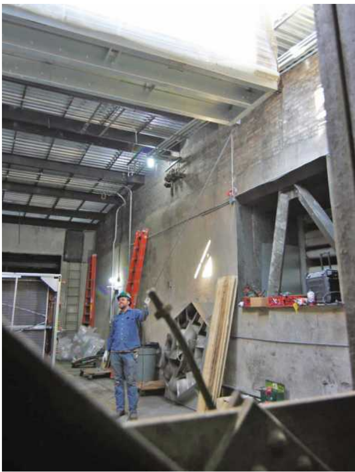
A PRESSURES AND PIPES worker guides the placement of HVAC equipment through the roof of the Frauenthal Center in Muskegon. Photo courtesy Pressures and Pipes
