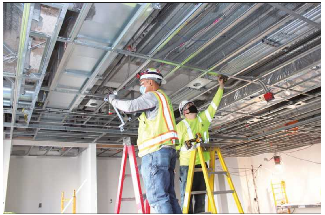
ELECTRICIANS Brian Lynch and Bill Wolfer of Local 58 work on lighting the second floor of the Olympia Development 2715 Woodward Building. They’re employed by Motor City Electric.
