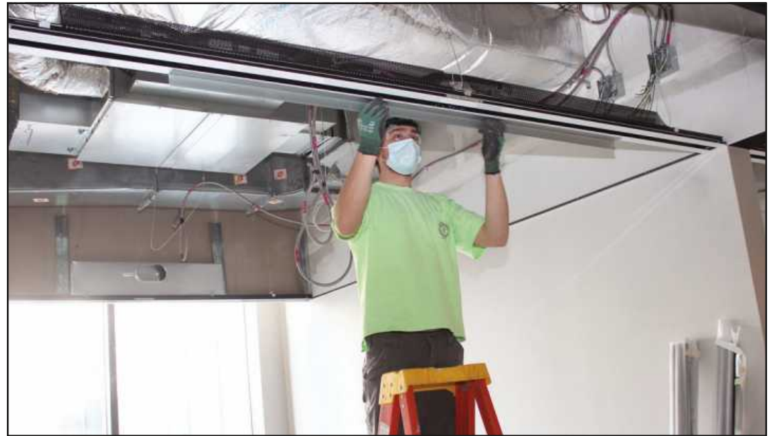
A LINEAR DIFFUSER is installed at the Olympia Development’s 2715 Woodward building by Ben Rudisill of Sheet Metal Workers Local 80. He’s employed by Dee Cramer.
