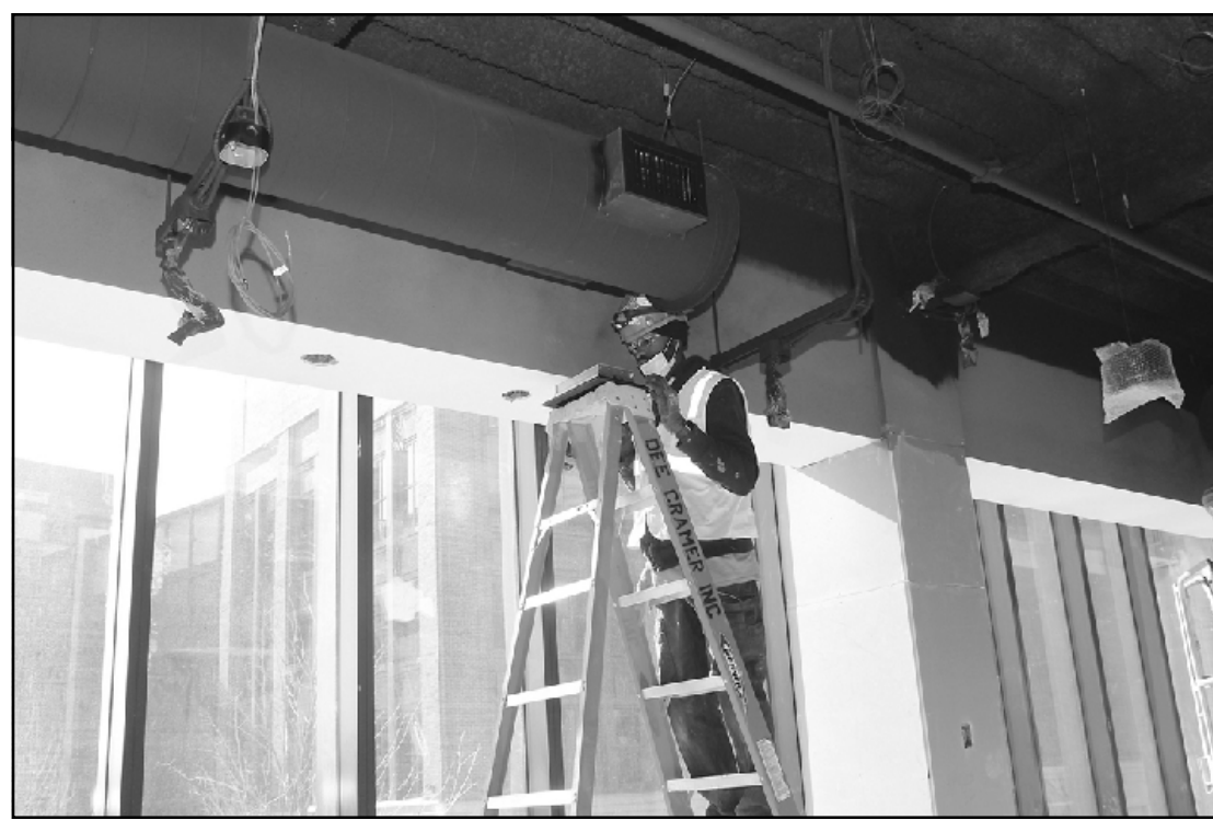
SETTING A DIFFUSER TAP for a mainline duct at the Olympia Development 2715 Woodward project in Detroit is Zarius Mayes of Sheet Metal Workers Local 80. He's employed by Dee Cramer.
