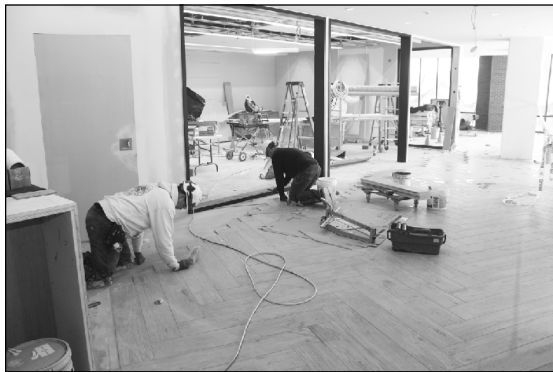
SETTING FLOORING on the third level of the Olympia Development's 2715 Woodward Building in Detroit are Bob Teague and Matt Suwinski of Bricklayers and Allied Craftworkers Local 2. They're employed by Empire Tile and Marble.
