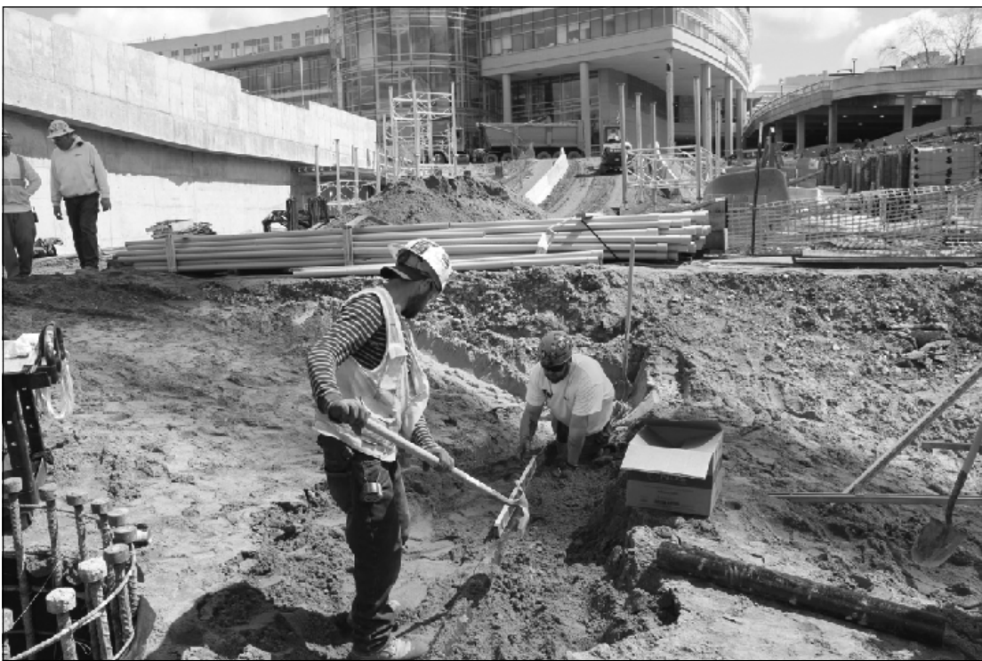
SETTING 4-INCH sanitary cast iron pipe at the University of Michigan Pavilion Health project in Ann Arbor are Dain Vettese and Justin Boughton of Plumbers and Pipe Fitters Local 190. They're employed by Boone and Darr.
