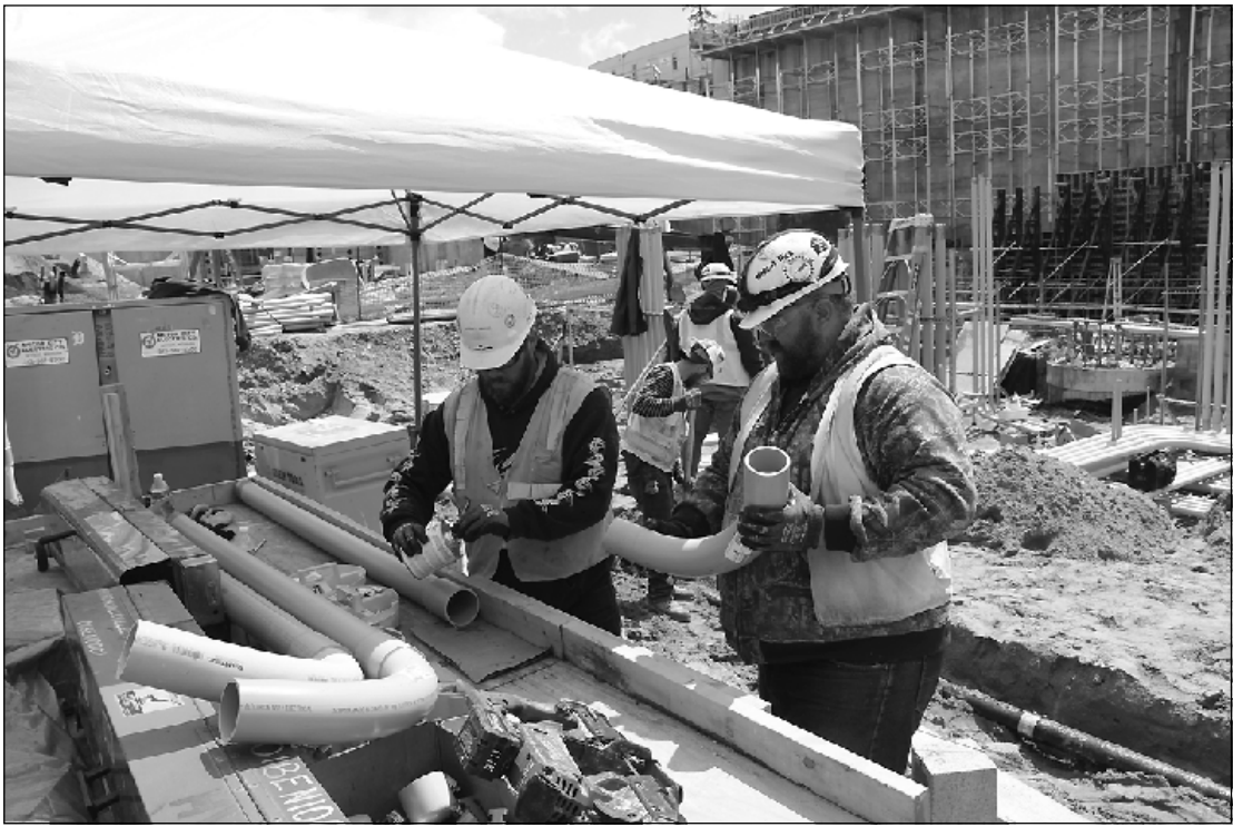
PIECING TOGETHER THREE-INCH PVC conduit at the University of Michigan Pavilion Health project in Ann Arbor are Andy Summers and Vic Tandy of IBEW Local 252. They're employed by Huron Valley Electric.
